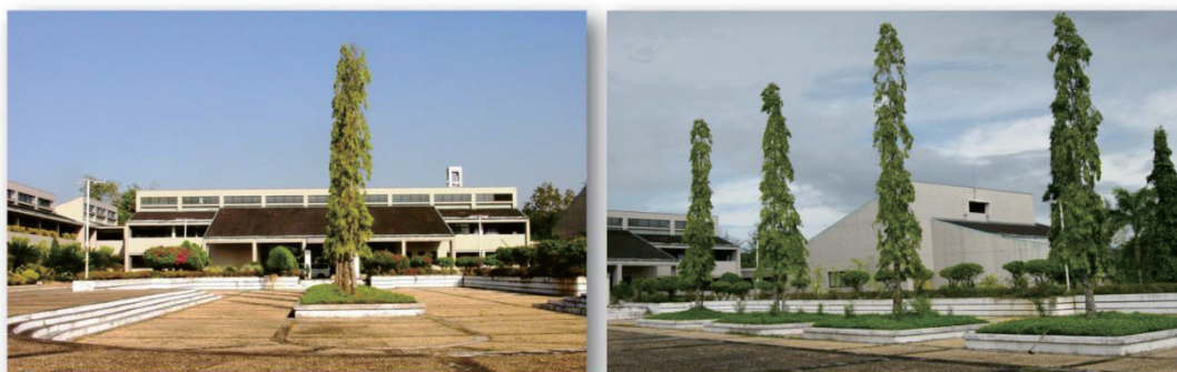
Figure 4-1-15.View of CFDTC main buildings
