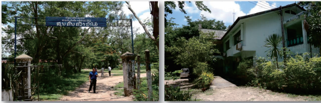
Figure 4-1-10. View of FSRC main building and main gate
