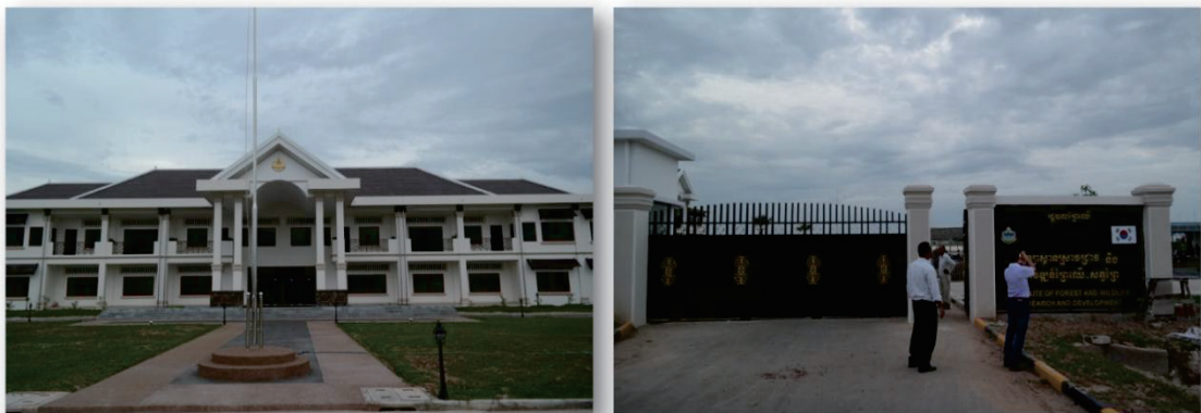
Figure 4-1-4. View of IRD main building and main gate
