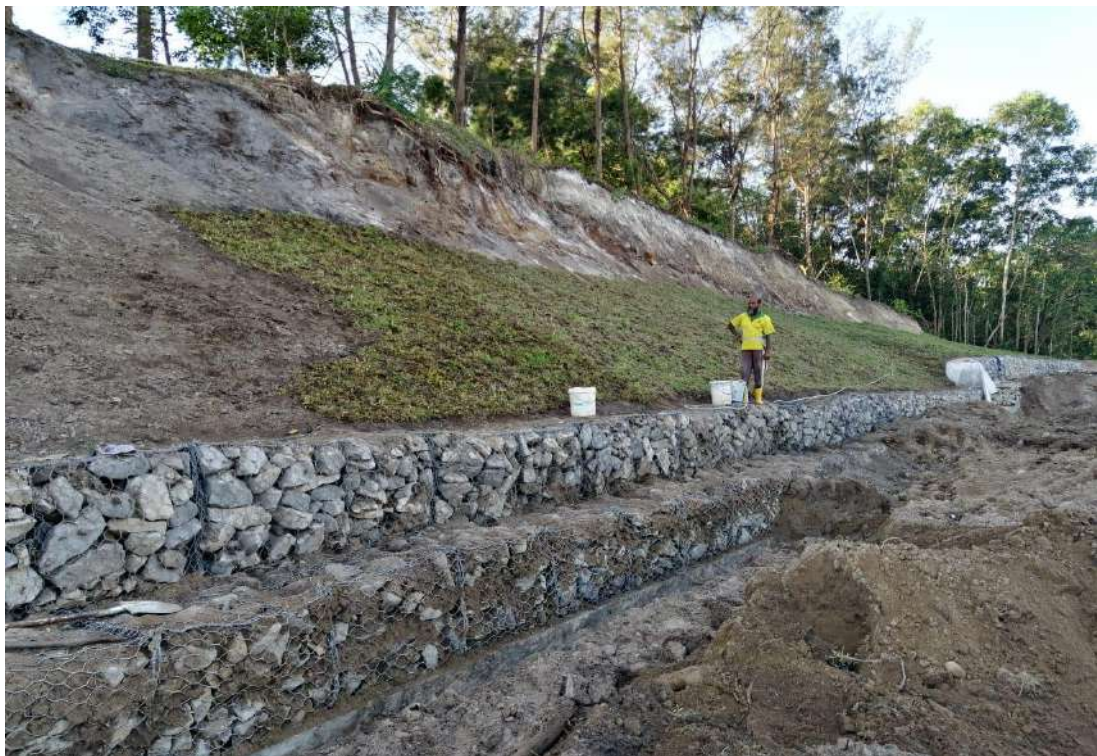
Slope and Gabion Wall
