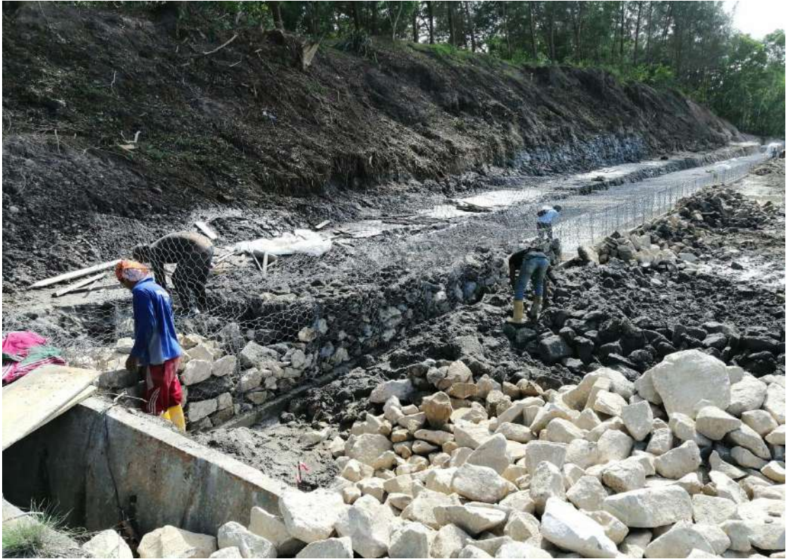
Slope Protection (Gabion Wall)
