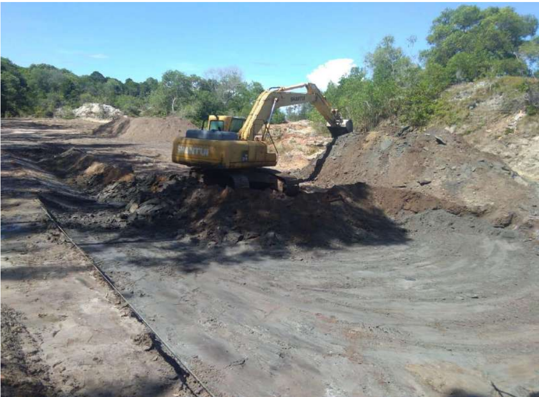
Levelling and backfilling
