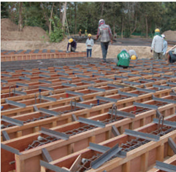
Construction work in December: Re-bar work for pile production
