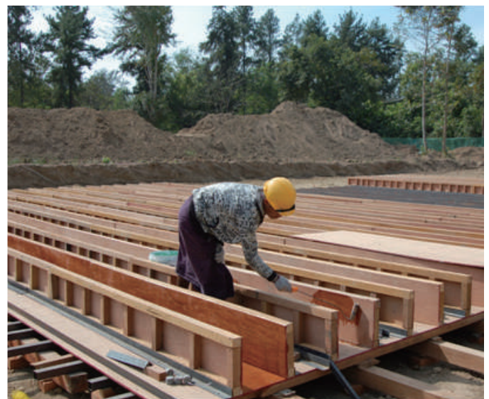
Construction work in December: Installation of casting molds for pile production
