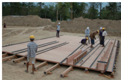
Construction work in December: Installation of casting molds for pile production
