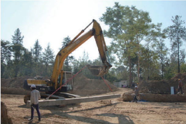
Construction work in December: Pile translocation to the target driving site
