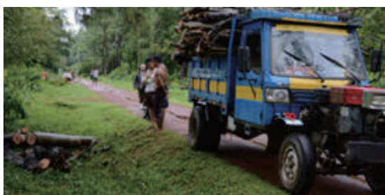
Tree logging and removal at the construction site for site clearance
