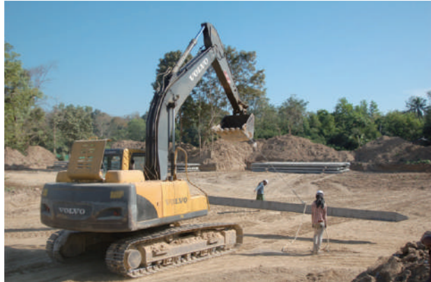
Construction work in December: Pile translocation to the target driving site
