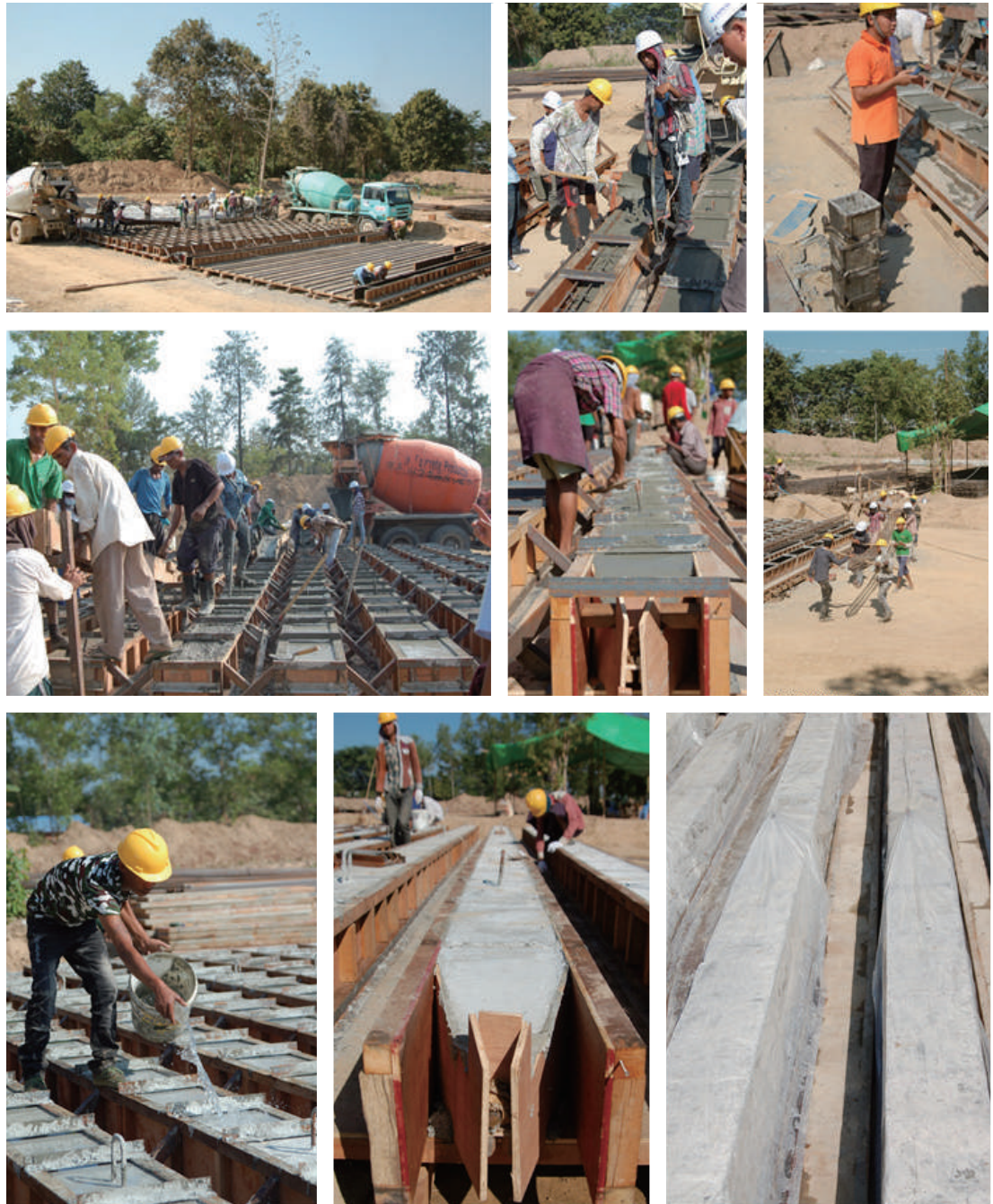
Construction work in December: Concrete casting and curing for pile production
